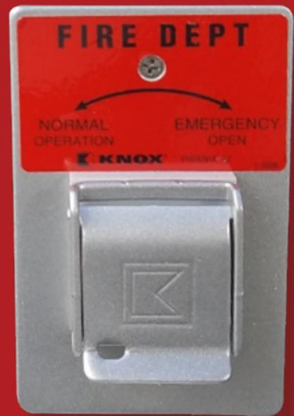
1. All occupancies served by Internal Automatic Fire Detection or Suppression System, having a connection to a Central or Remote Station Monitoring Facility, shall be provided with a Knox Access Box. The Knox Access Box must be approved by the Office of the Fire Marshal
